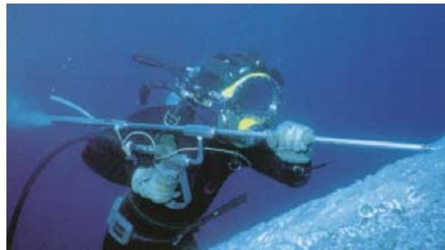
Underwater washing/sandblasting for NDT inspections, hull washing, thermoelectric power plants sea-line cleaning, underwater piping and line maintenance, wreckage recoveries (underwater archaeology).
